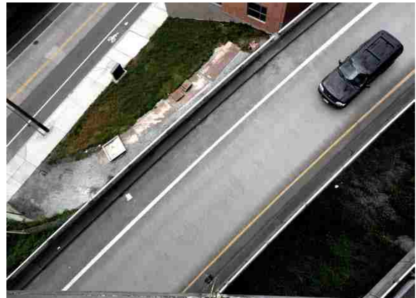
figure 17: View from Lakeview overpass
