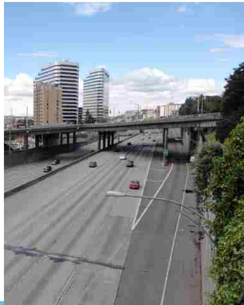
figure 49: maps and image of the first site on the spine trail starting from the south end
